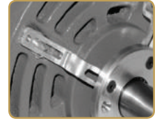
AEGIS® EP2400 Conductive Epoxy installation
